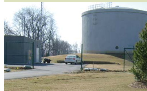
The storage tank and booster station located on River Road in Sterling provides an additional 500,000 gallons of capacity as well as enhances water pressure and fire protection.
