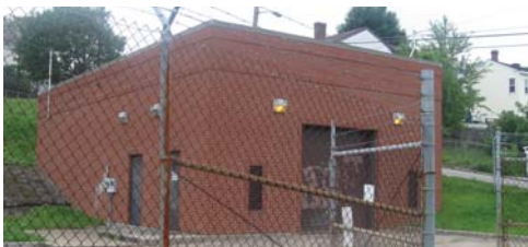
The Arlington Booster Station will be receiving new chemical storage and feed facilities.
