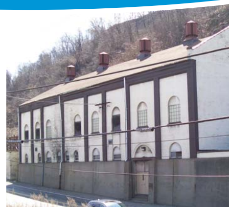
The existing Becks Run raw water pump station was constructed in 1894 and has been upgraded numerous times.
