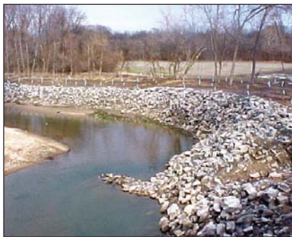
Piasa Creek Watershed improvements began in 2001 and have included numerous projects such as rock stabilization of a streambank that prevents erosion and creates pools and riffles for fish (left). Construction of stream barbs helps to reduce erosion and improve fish habitat (right).
