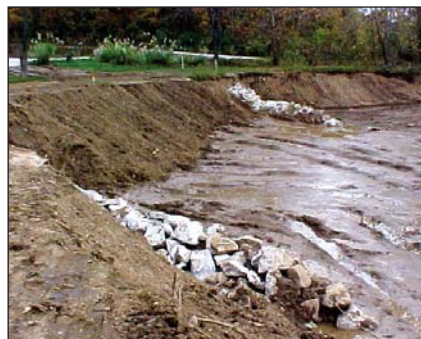
Piasa Creek Watershed improvements began in 2001 and have included numerous projects such as rock stabilization of a streambank that prevents erosion and creates pools and riffles for fish (left). Construction of stream barbs helps to reduce erosion and improve fish habitat (right).
