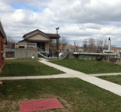
Fairview wastewater treatment plant
