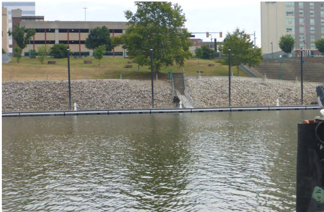
Figure 11: Typical bank protection along the Charleston Waterfront.
