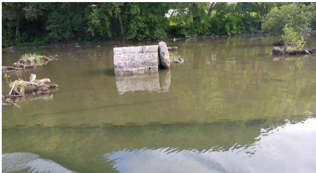
Figure 22: Timber sheeting and shallow area near the north bank.
