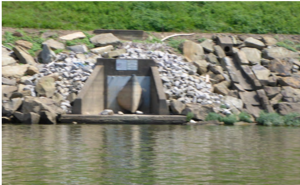
Figure 13: Large outfall pipe along the Charleston Waterfront.
