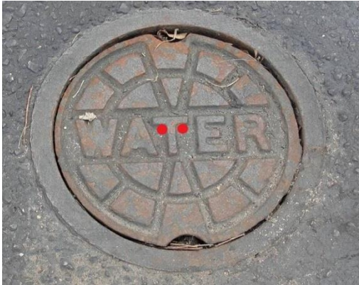
Figure 1. The red dots show the standard locations for position of the central pole point.
